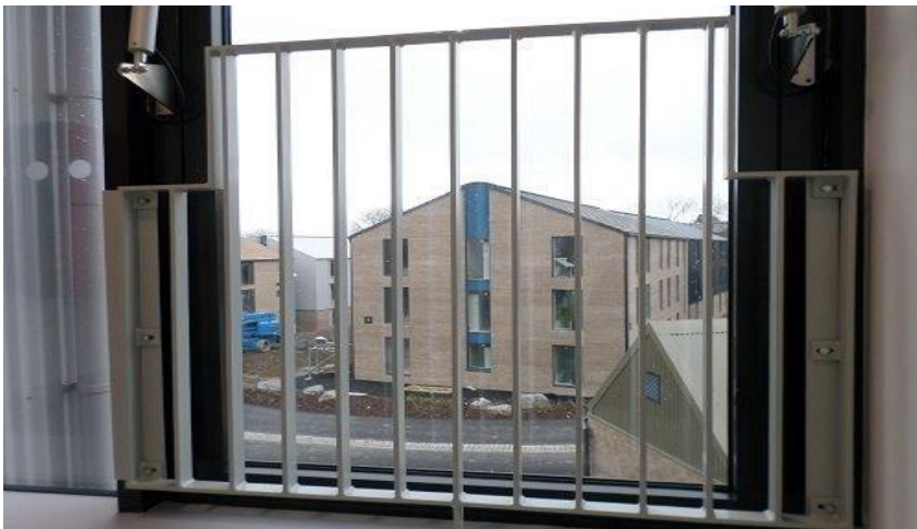
Effective protection for Juliet balconies in the student accommodation.
