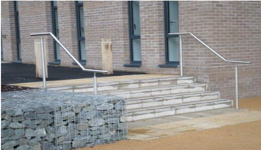
Simple stainless steel handrails are both practical and visually pleasing.
